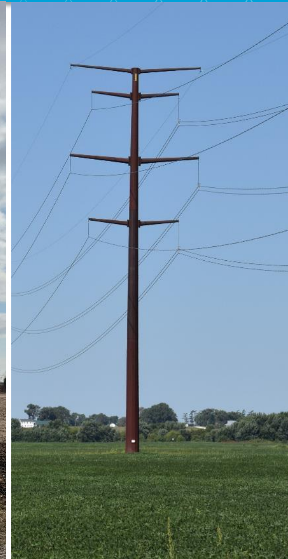
New steel monopole structure
