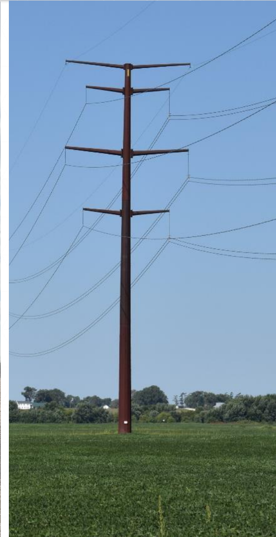
New steel monopole structure
